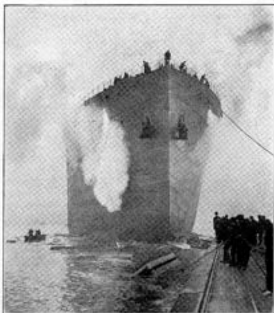
The Belgeland Just After Launching
